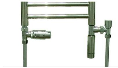
This combination allows you to have control whilst the central heating is on and when you use the element. The lockshield valve does not fit under the bottom bar so has to go on the outside of the rail.
